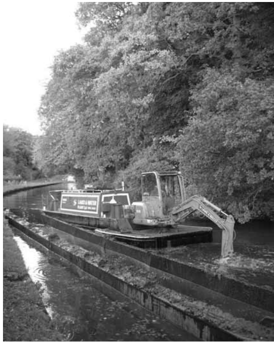
Figure 23.4 Dredger on floating barge
