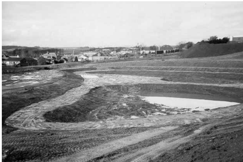
Figure 21.1 A pond under construction
