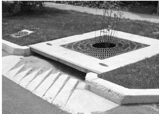
Figure 19.8 Highway inlet deflector system (courtesy Robert Bray Associates)
