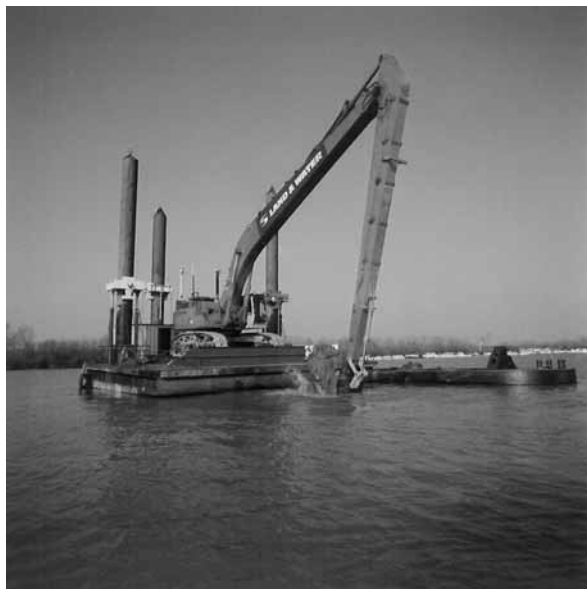
Figure 23.5 Long reach excavator on floating pontoon
