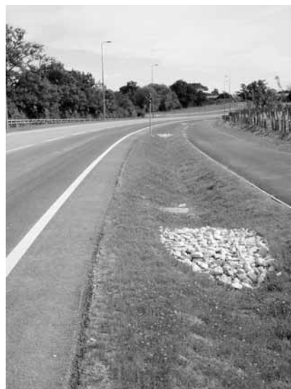
Figure 10.5 A check dam
