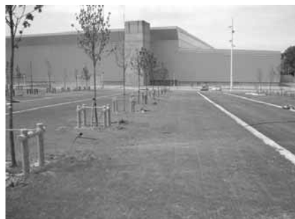
Figure 12.3 Green pervious pavement systems
