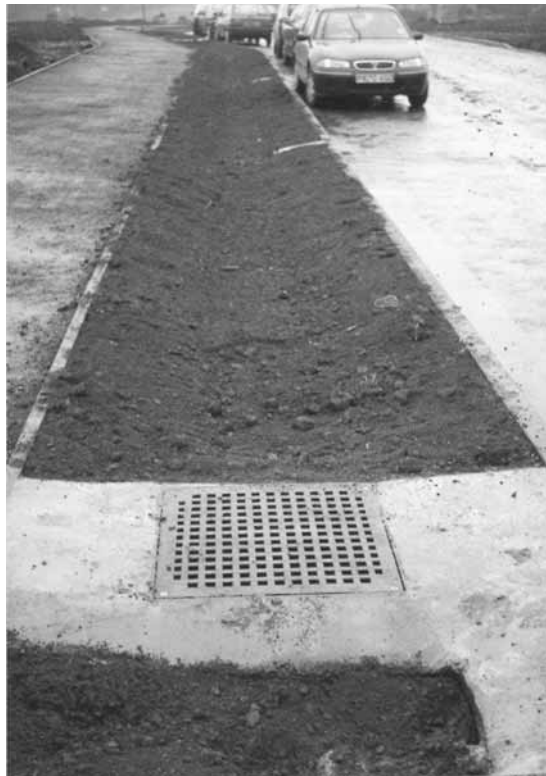
Figure 21.2 Construction of a swale
