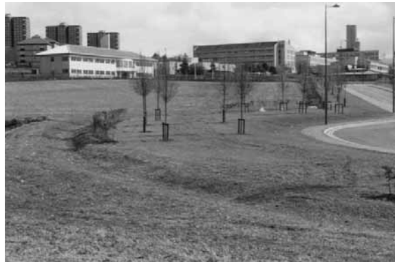
Figure A2.4 Conveyance swale
