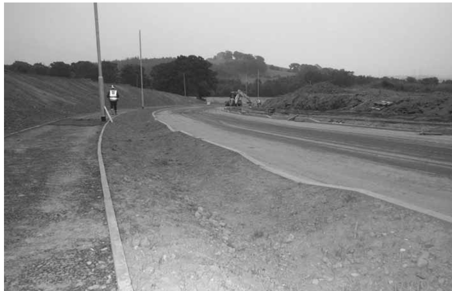
Figure 21.5 A swale under construction
