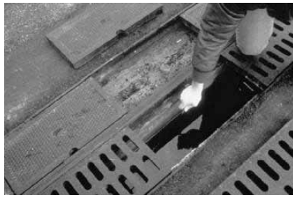
Figure 14.3 Perimeter sand filter
