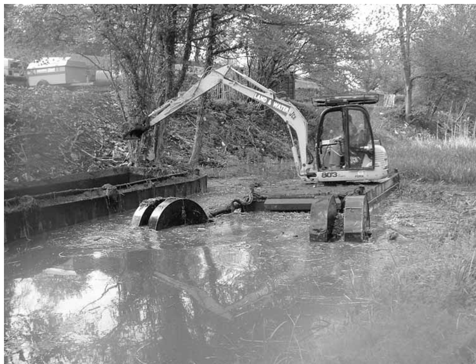
Figure 23.3 Floating excavator working in small pond
