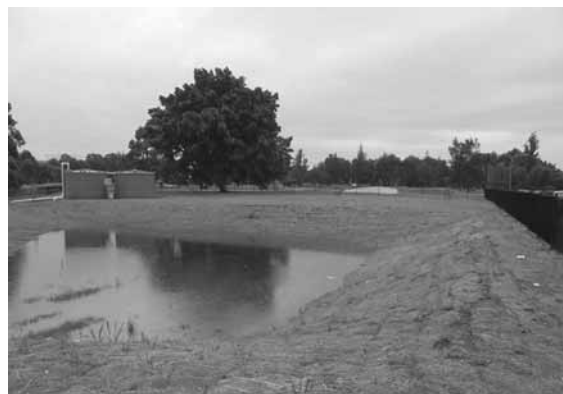
Figure 14.1 Surface sand filter
